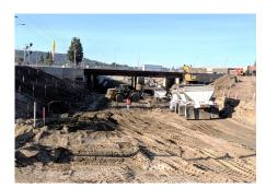
**Puente Avenue Grade Separation Project...** This project will provide a new roadway underpass on Puente Avenue and Workman Mill Road, with new bridges built for the Union Pacific Railroad and Valley Boulevard. A loop connector road has reestablished connectivity between Workman Mill Road and Valley Boulevard. This project is 75 percent complete, with the new roadway expected to open to traffic in April 2018 and full project completion in January 2019.
