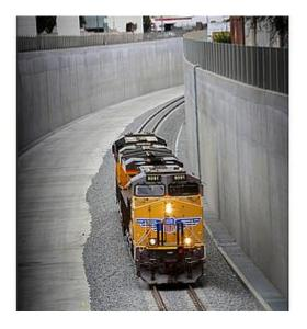
USA: A 2-3 km long, 9 m deep and 20 m wide cutting built at cost of \$313m as part of a grade separation project designed to ease traffic congestion in the San Gabriel Valley east of downtown Los Angeles was officially opened by the Alameda Corridor-East Construction Authority on July 24, eliminating four level crossings.
