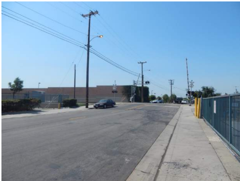
Photograph 2: View along S. Maple Avenue facing south from north of the Union Pacific Railroad
