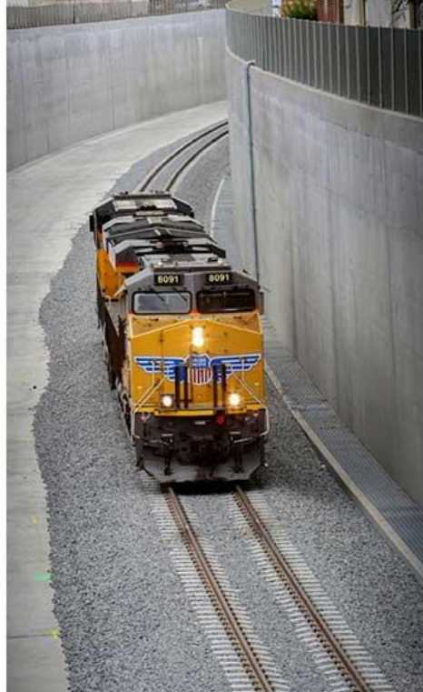
Trains have started rolling on the new $313 million San Gabriel Railroad Trench (photo courtesy of ACE)
