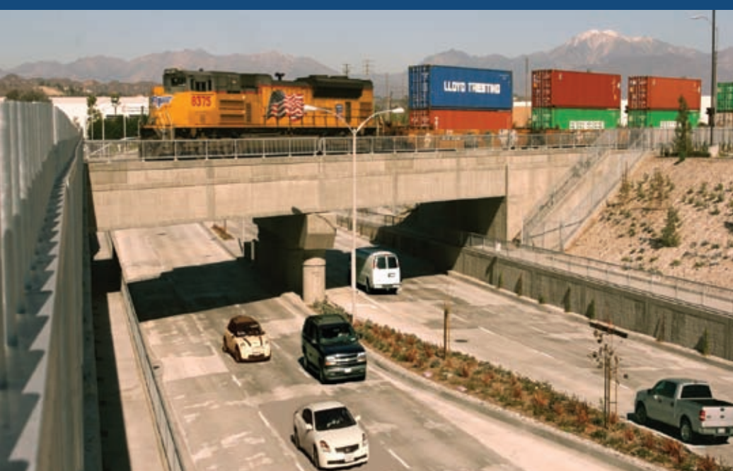
The busy Brea Canyon Road grade separation project in the Cities of Diamond Bar and Industry is used daily by 21,000 motorists, three-dozen freight trains and over a dozen commuter trains.
