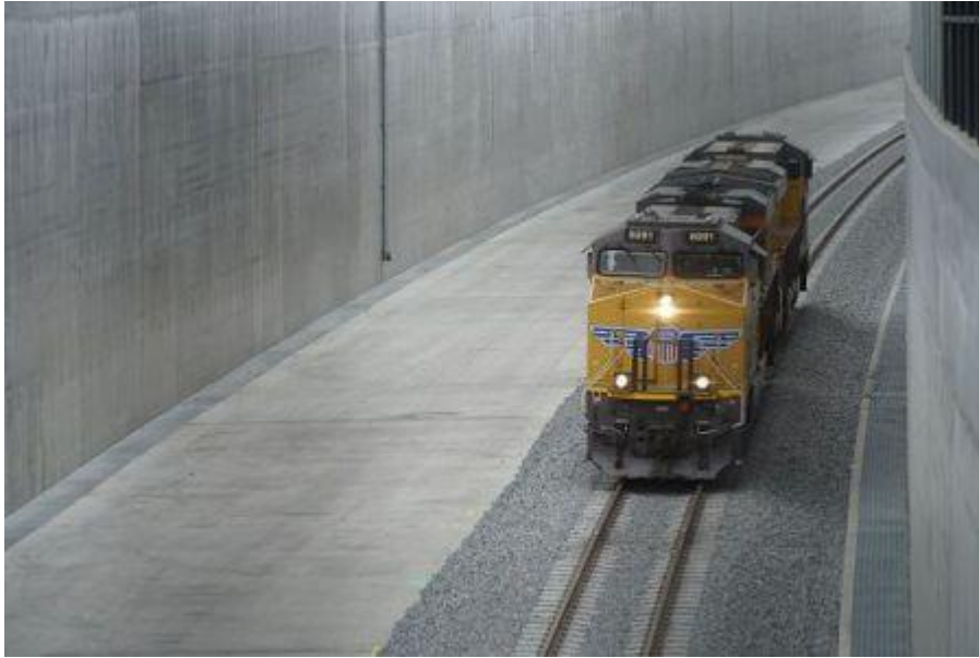
Inaugural train service runs through San Gabriel trench. City of San Gabriel
