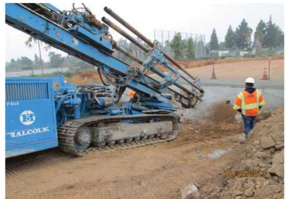
*SGT Retaining Wall Tie Back Testing and Installation*
