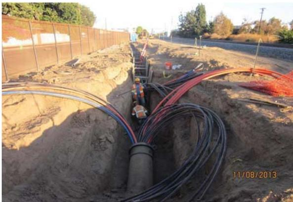
*SGT Fiber Optic Cable Pulling and Splicing*
