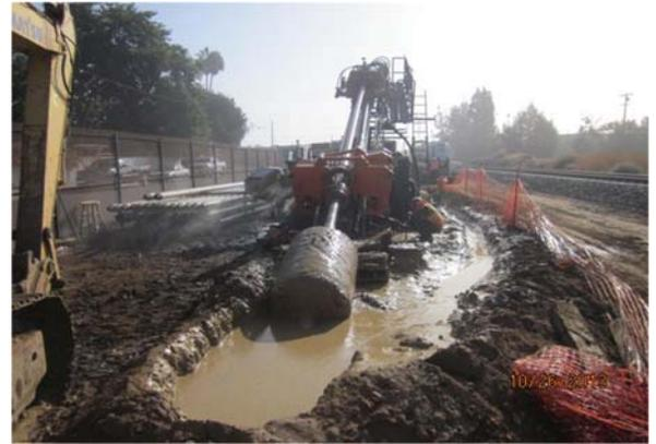
*SGTC Fiber Optic Installation Drilling*
