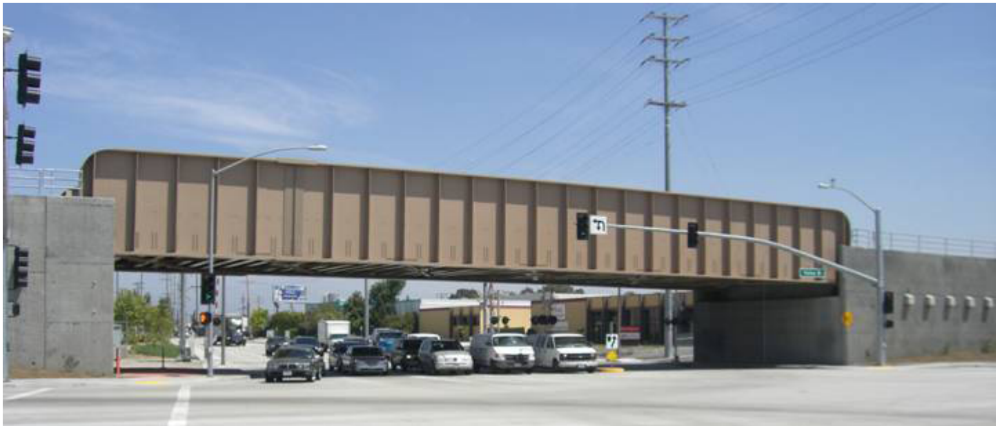
View of completed Sunset Avenue railroad bridge looking north from Valley Boulevard
