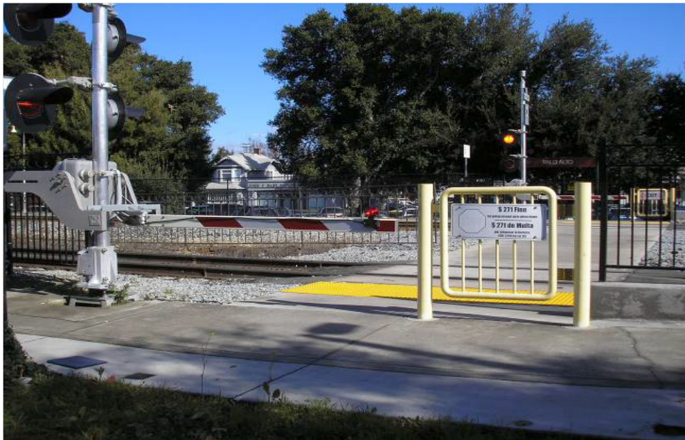
Image of the type of pedestrian gates proposed for installation at Pomona rail crossings.
