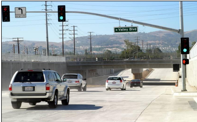
At left, view of completed Valley Boulevard bridge and railroad bridge on southbound Nogales Street.
