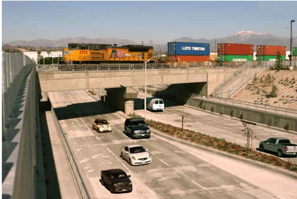
Completed Brea Canyon Road Grade Separation
