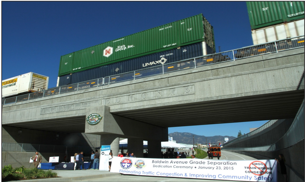
Completed grade separation project. View looking north on Baldwin Avenue.
