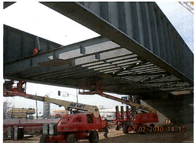
Erecting Sunset Ave Floor Beams
