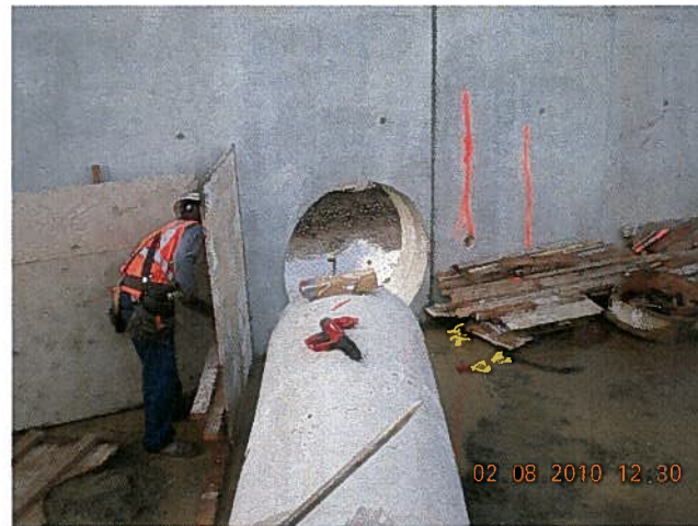
Constructing Drainage Line " Through Main Track RW
