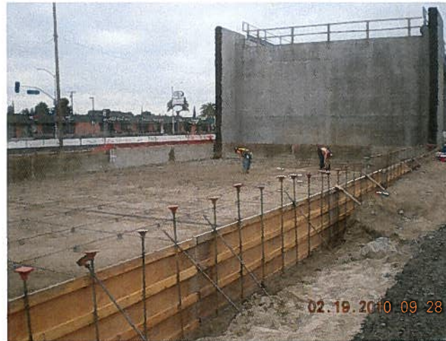
Forming Orange Abutment 2 Footing
