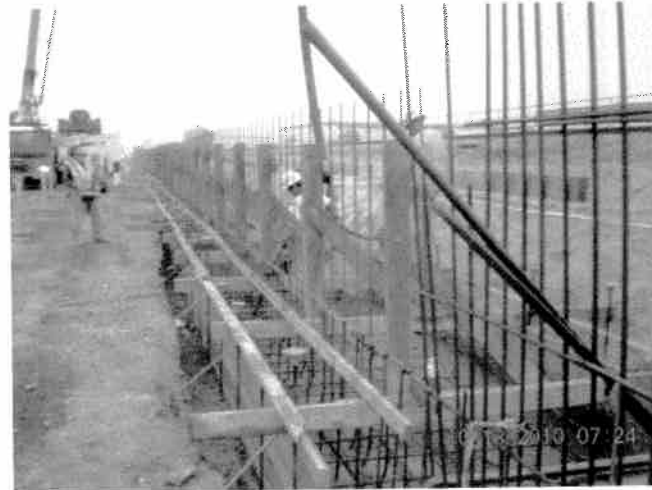
Formed & Poured Remaining Retaining Walls for ML Track
