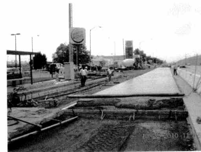
PCC Paving on Eastbound Valley Blvd.
