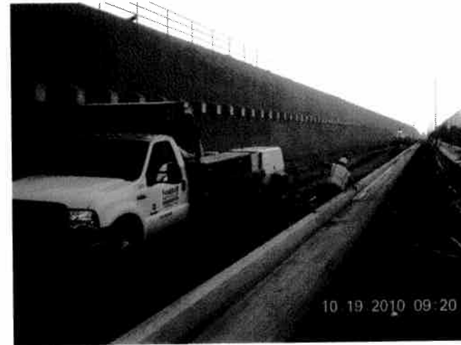
Valley Blvd Curb & Gutter
