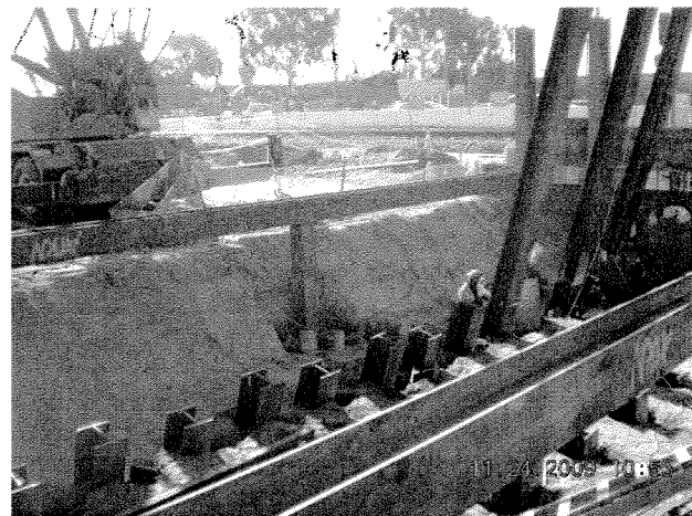
Pile Driving Battered Piles at Sunset Abutment
