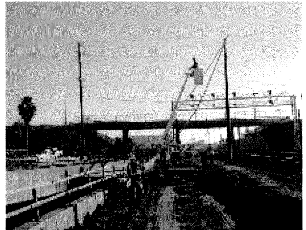
Final Relocation of MCI Fiberline
