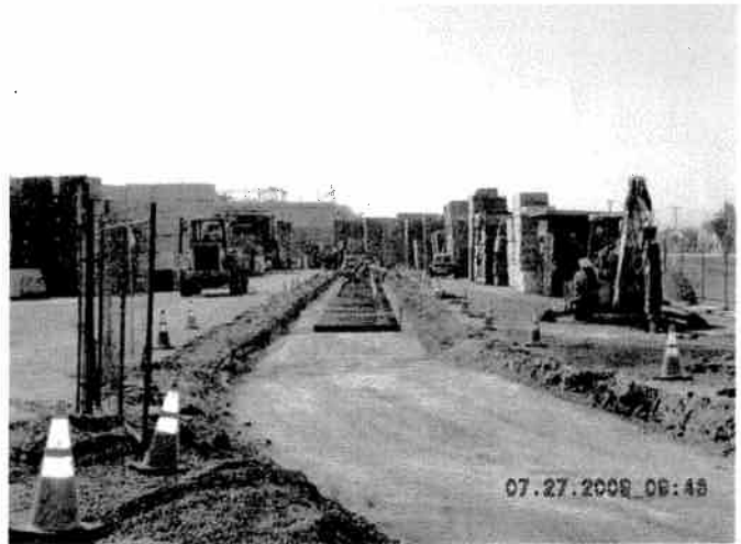
Spur 858 Construction (CN 050)
