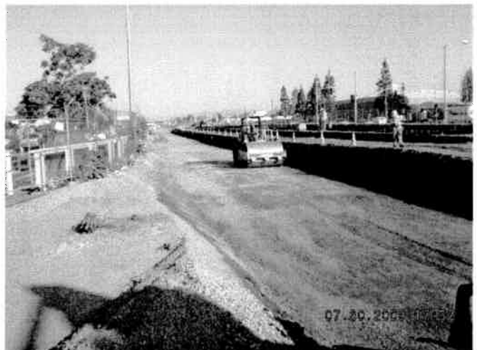
Drill Track Stage 3 Over-Excavation
