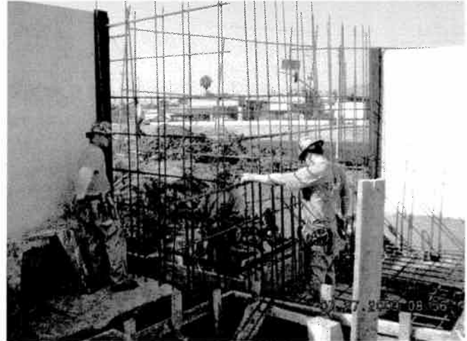
Installing Rebar for Fresh Point RW (CN 039)
