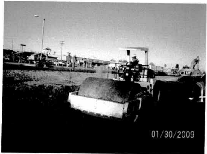
Drill Track Grading (CN 025)
