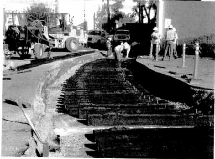
LA CORR Spur 861 Work
